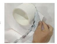
5. With the flashing still folded at the crease, extend length of DuPont™ FlexWrap™ EZ and gently remove remaining release paper. Avoid stretching DuPont™ FlexWrap™ EZ.
