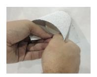
8. Fold the second piece of DuPont™ FlexWrap™ EZ to break perforations in release paper and create a sharp crease. Remove narrow (~1") width of release paper. While still folded, center DuPont™ FlexWrap™ EZ above the pipe and use the remaining release paper to position tight against the WRB. Adhere the exposed butyl to the top, and down each side of the pipe to the 3 and 9 o'clock positions.
