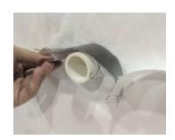
10. Position the unadhered butyl of the narrow section below to overlap the edges of DuPont™ FlexWrap™ EZ installed first by a minimum of 1". Use thumbs to adhere. Do not stretch DuPont™ FlexWrap™ EZ.
