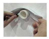
9. Extend the length of DuPont™ FlexWrap™ EZ and gently remove remaining release paper to avoid stretching the product.
