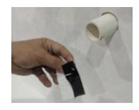
4. While still folded, center DuPont™ FlexWrap™ EZ under the pipe and use the remaining release paper edge to position DuPont™ FlexWrap™ EZ tight against the WRB. Adhere the exposed butyl to the underside of the pipe.
