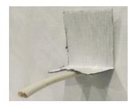
5. Extend both sides of DuPont<sup>™</sup> FlexWrap<sup>™</sup> EZ below the wire and adhere each corner and outside edge to WRB as shown.
