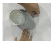
8. Fan out the remaining DuPont™ FlexWrap™ EZ onto the WRB around the circumference of the pipe. Use firm hand pressure on both pipe and WRB surfaces for a good bond and a secure seal. If any wrinkles or creases form during application, ensure they are smoothed out and adhered with firm hand pressure.
