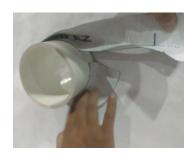
7. Unfold and fan out DuPont™ FlexWrap™ EZ applied at the 3 o'clock position to the WRB. Adhere the remaining exposed butyl of DuPont™ FlexWrap™ EZ to lap over the layer below and then onto the WRB.
