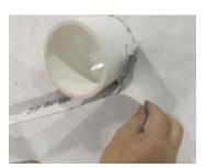
6. Continue to adhere DuPont™ FlexWrap™ EZ around the circumference of the pipe to the 1 o'clock position by gently placing the exposed butyl onto the pipe surface with minimal tension.
