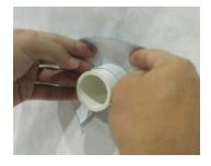
**12.** Use firm hand pressure on both pipe and WRB surfaces for a good bond and secure seal. Remove any wrinkles or creases by using firm hand pressure to ensure a fully adhered and smooth surface.
