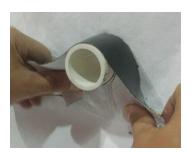
Fan out the remaining unadhered DuPont™ FlexWrap™ EZ onto the WRB above and down each side of the pipe.
