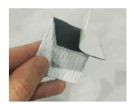
4. Position DuPont™ FlexWrap™ EZ above the wire so the exposed butyl is centered on top of the wire, and the side with remaining release paper is against the WRB.
