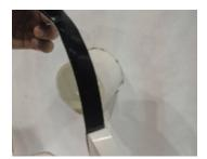
4. With the flashing still folded at the crease, use the remaining release paper edge to position DuPont™ FlexWrap™ EZ tight against the WRB at the 3 o'clock position and adhere a small section of the exposed butyl onto the pipe.
