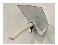
6. Pinch together the exposed butyl of DuPont™ FlexWrap™ EZ below wire to create a flap and complete a full perimeter seal around wire. Use firm hand pressure to remove any pinholes at the crease below the wire where the butyl is adhered together.
