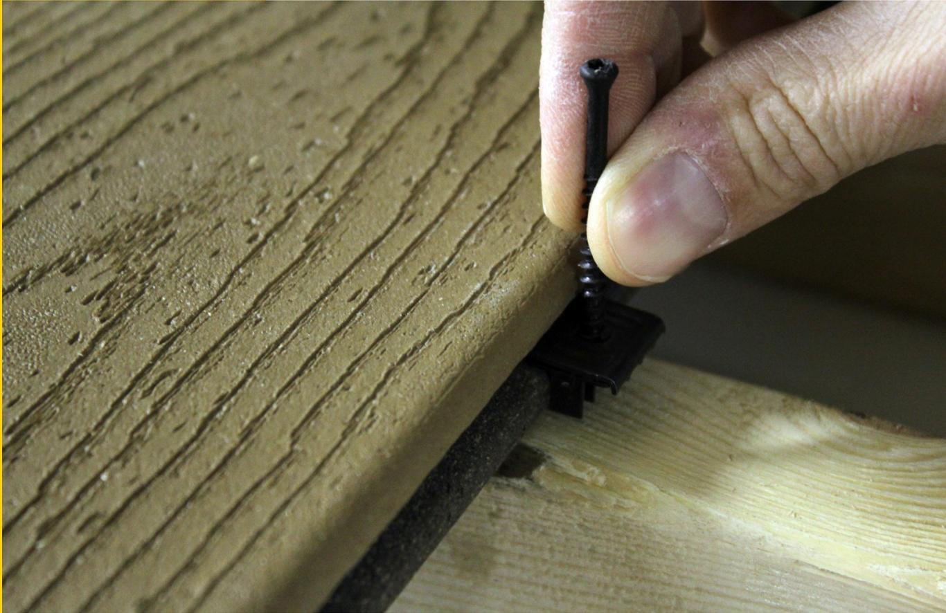
**CAMO Clips are universal hidden fasteners that have incredible versatility to work with most grooved deck boards including Trex®, TimberTech®, AZEK®, Fiberon and many more, delivering a beautiful fastener-free deck top. The black oxide coating and stainless steel construction gives you excellent corrosion resistance. The CAMO Clips Limited Warranty gives you the security to relax and enjoy your deck.**
