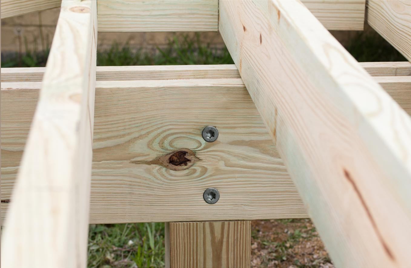
**From deck substructure to landscape timbers, CAMO multi-purpose structural and ledger screws are an easy, code compliant way to replace 3/8" (10mm) and 1/2" (13mm) lag screws.**
