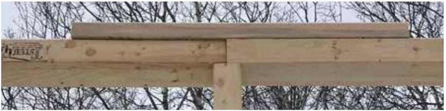
Temporary blocking used as a stiffener when standing up the wall.
