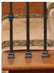
Open Tread Bottom Connection
