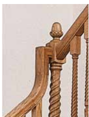
Landing Fitting Assembly (gooseneck) is used with a short block newel post at all landings.
