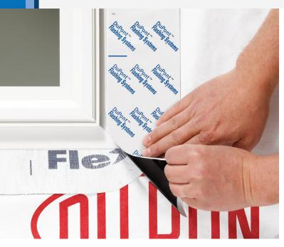
DuPont™ Flashing Tape is easy to install with a forgiving initial tack.
