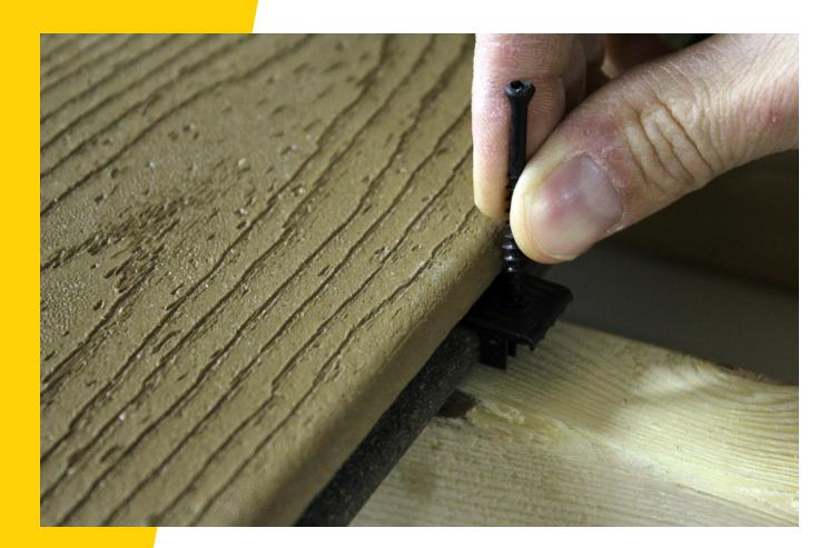
CAMO Clips are universal hidden fasteners that have incredible versatility to work with most grooved deck boards including Trex®, TimberTech®, AZEK®, Fiberon and many more, delivering a beautiful fastener-free deck top. The black oxide coating and stainless steel construction gives you excellent corrosion resistance. The CAMO Clips Limited Warranty gives you the security to relax and enjoy your deck.
