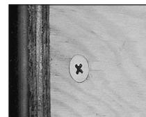
Plywood to steel or wood studs.
